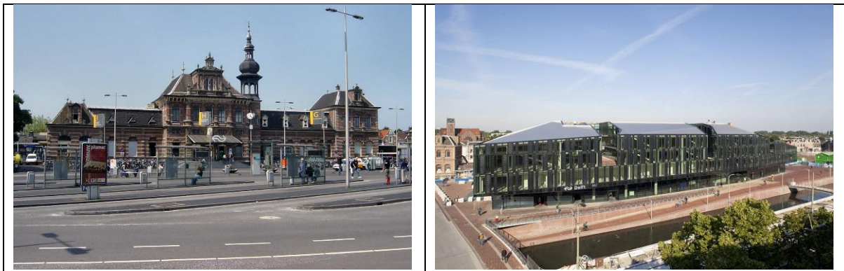
Figure 1: Delft Railway station before (left) and after (right) redevelopment
