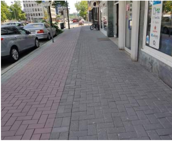
(c) Textural separation, cyclists could swerve onto the sidewalk, Nuremberg.
