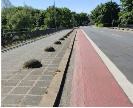
(b) Structural separation with curb, Nuremberg.
