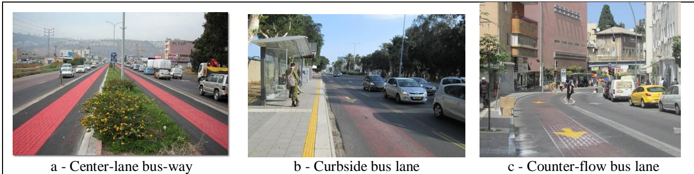
Figure 1. Examples of bus lane configurations in Haifa BRT system.
